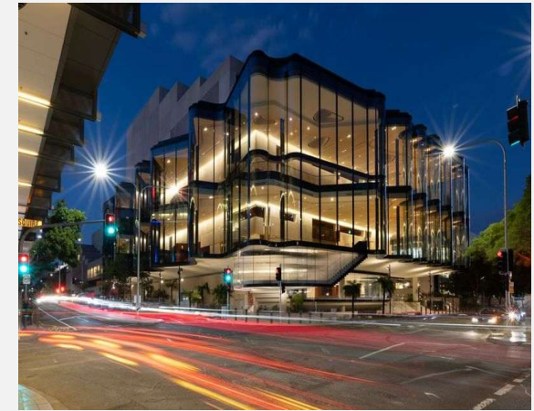
Glasshouse Theatre, South Brisbane Photograph Credit : David Kelly
