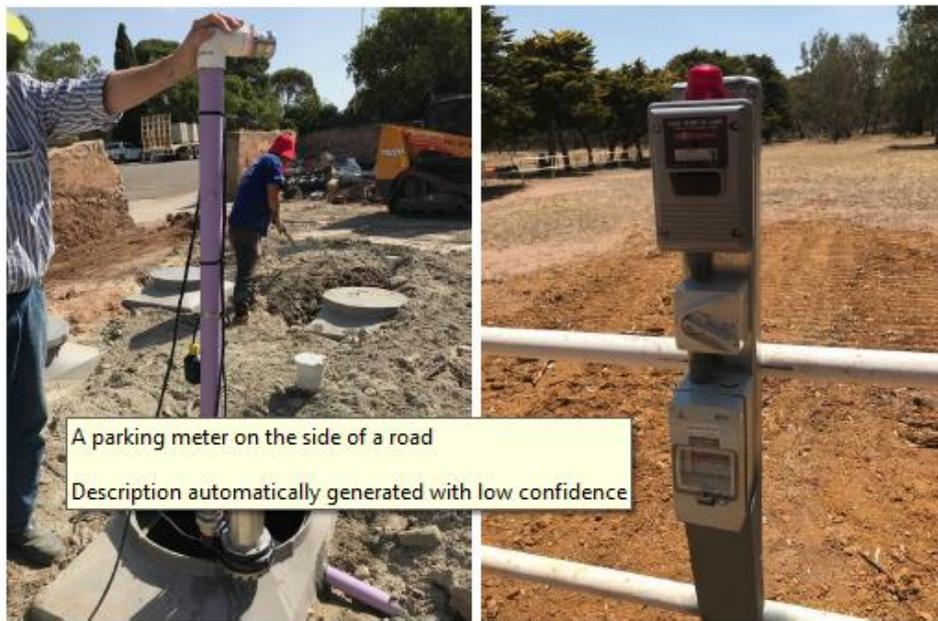
Figure 5 Typical Pump and alarm panel installation showing circuit breaker and isolation switch
