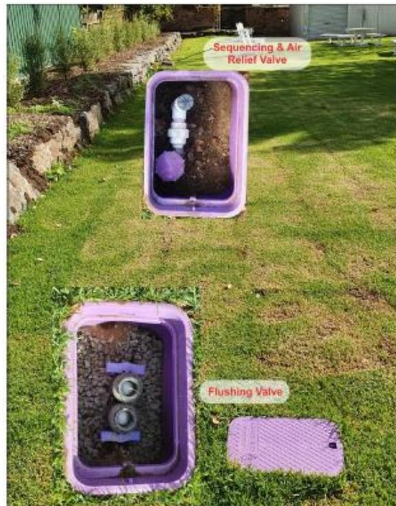
Figure 7 ABSORBS™ system showing valve boxes with sequencing, air relief and flushing valves
