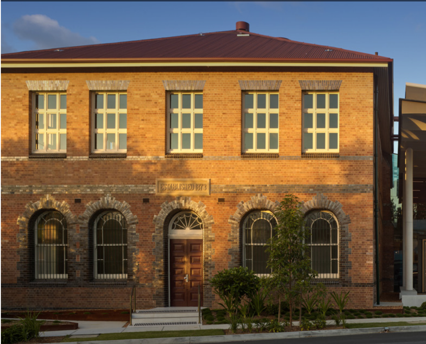
The Thomas Dixon Centre, Home of Queensland Ballet by Conrad Gargett. Photographer: Christopher Frederick Jones.
