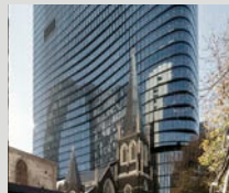
Wesley Place Precinct. COX Architecture, Lovell Chen, Oculus. Photographer: Lynton Crabb, Trevor Mein. Client: Charter Hall, Uniting Church
