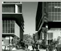
A1 @ SW1, SOUTH BANK Cox Architecture and Gamble McKinnon Green, Christopher Frederick Jones
