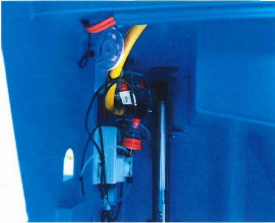
Chlorinator automatically doses chlorine through flow rate to the required amount
