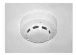
Early warning systems (fire alarms) for budget accommodation buildings can range from self contained smoke alarms (such as 240Volt AC mains powered) through to commercial smoke detection systems connected to the fire service.
