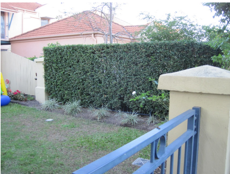
Acceptable – vegetation too dense to allow for climbing.
