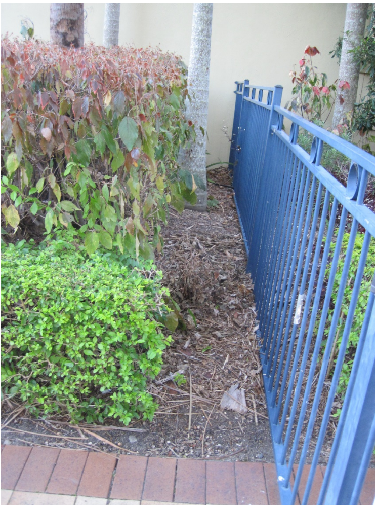
Acceptable – vegetation removed from the inside cleared area.
