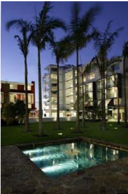
Lot 14 (The Village Centre) at KGUV incorporates a planted roof and recreation area for residents over the shopping centre component of the project.
