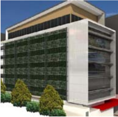
Lots 30 + 31 at KGUV provides an example of how a green wall can be used to improve sunshading, privacy and amenity.
