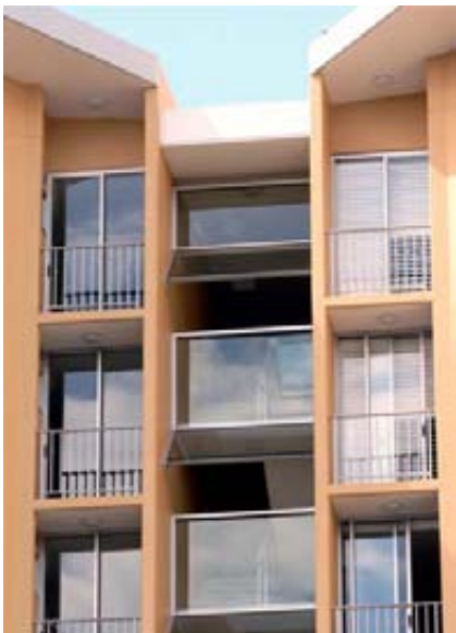
Naturally ventilated apartments via stairs and lobbies at the Village Centre (Lot 14 KGUV).
